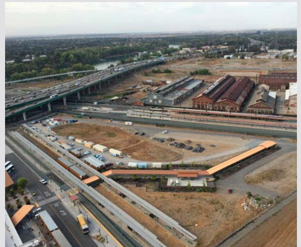
The 19th century brick buildings, originally called the Central Shops, will be incorporated into future Sacramento Yard development.
