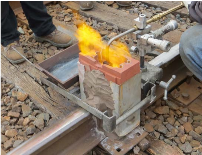
Internal rail flaws are repaired without removing an entire section of rail with thermite head repair welding technology. This lowers the risk of rail defects in the track repair process.
