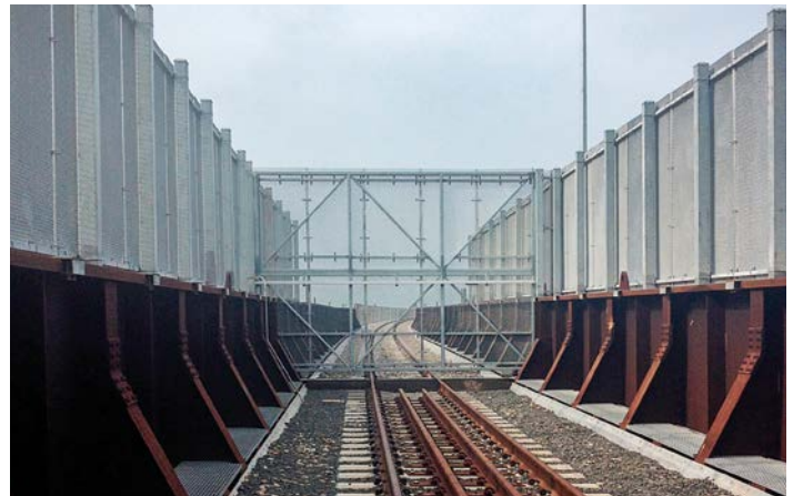
The West Rail Bridge connecting Brownsville, Texas, and Matamoros, Tamaulipas, Mexico, is the first international rail bridge built in more than a century.
