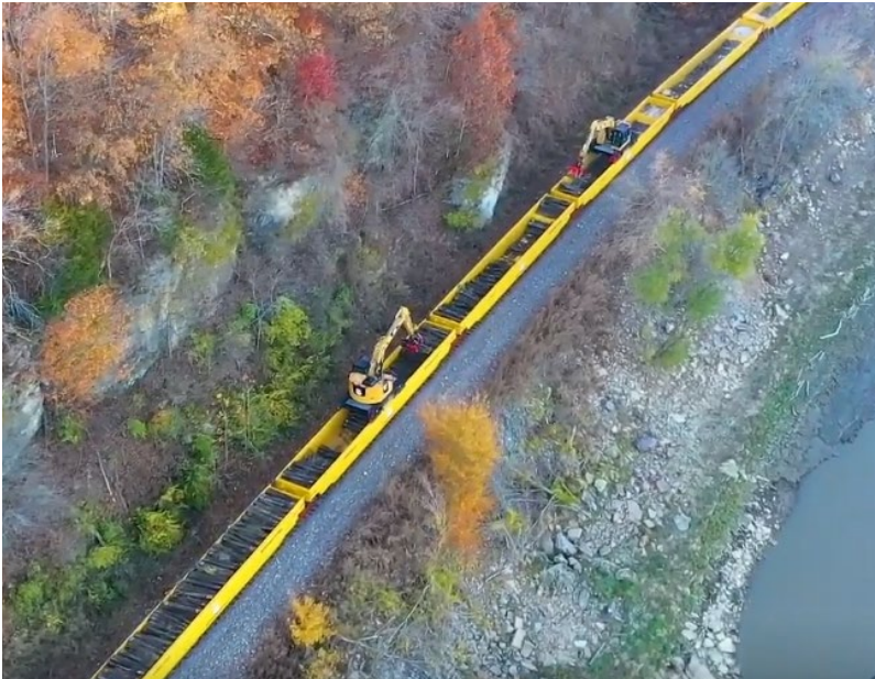
We are speeding up our used rail tie pickup process with specially designed work equipment to enhance safety and efficiency. We annually divert 90% of our used railroad ties away from landfills to energy recovery facilities.
