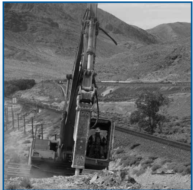
Hydraulic impact hammer "Hoe-Ram" breaking rock in preparation of installing conduit
