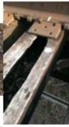
Treating plants sometimes get the kerf on the wrong side, heartwood, and if large checks and splits appear on that side, flip the tie over to the sapwood side, which is free of large check/splits and install up.
