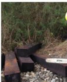
*Field cuts are made to wood timbers out of necessity, yet they breach the treated layer of wood and open up a pathway for fungi and insects. Recovering the cut area with preservative will seal it and prevent decay.*
